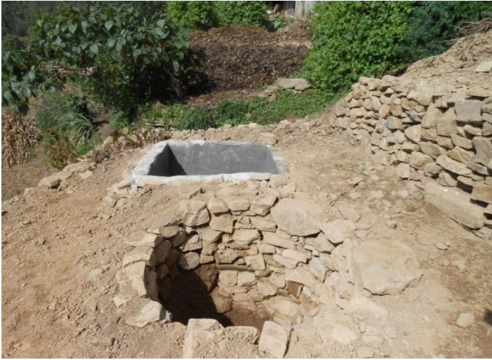
Bio-char pit to produce organic fertilizer
